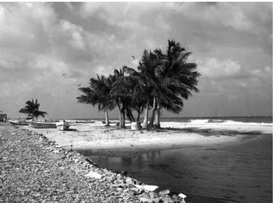
Coastal road under reconstruction, Mullaittivu, December 2005
